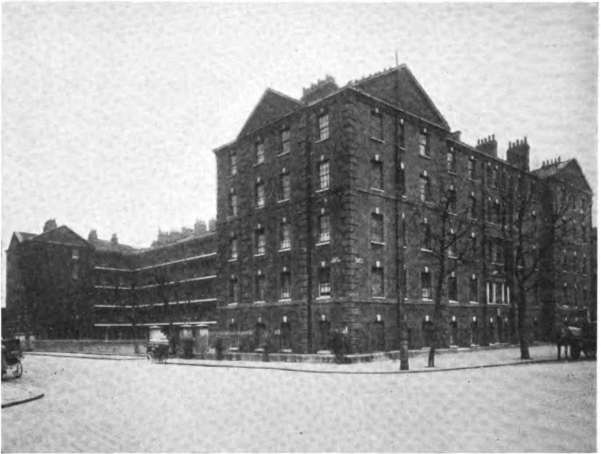
DWELLINGS ERECTED IN 1846 BY THE METROPOLITAN ASSOCIATION
