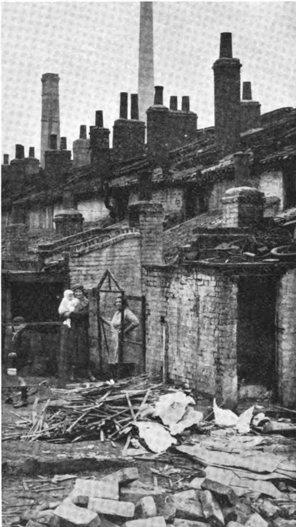
HOUSES IN THE VAUBAN STREET AREA—BEFORE CLEARANCE BY BERMONDSEY METROPOLITAN BOROUGH COUNCIL
