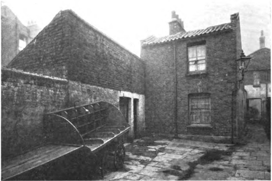
CHINA WALK AREA—VIEW, BEFORE CLEARANCE, OF KARL PLACE
