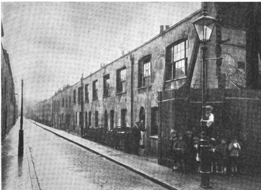
WARE STREET AREA—VIEW, BEFORE CLEARANCE, OF MILL ROW
