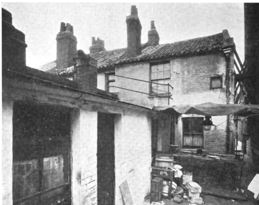
WYNDHAM ROAD AREA—VIEW, BEFORE CLEARANCE, OF 46, WYNDHAM ROAD
