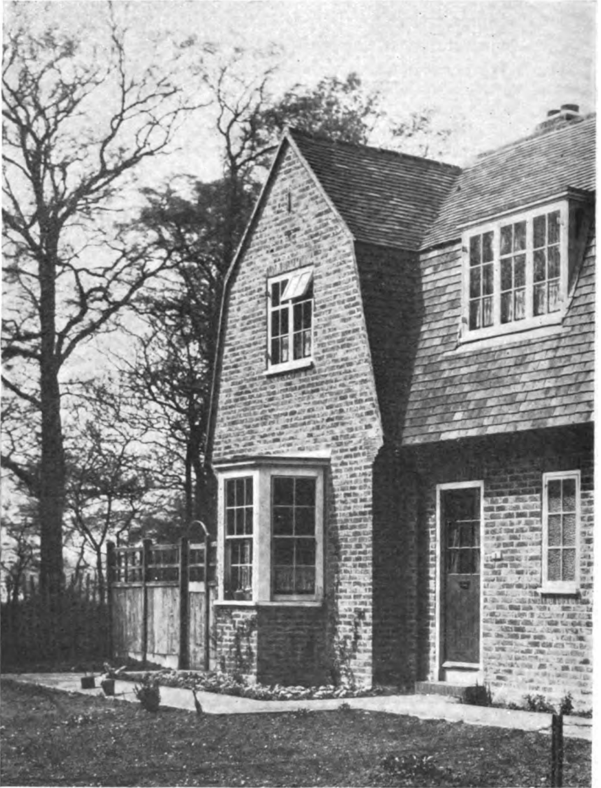
DOWNHAM—NO. 9, DOWDERRY ROAD
