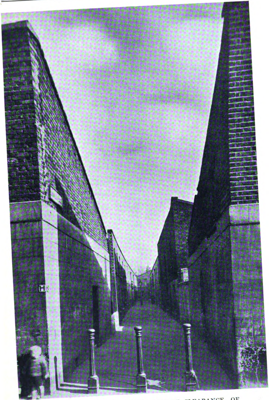
TARN STREET AREA—VIEW, BEFORE CLEARANCE, OF LINWOOD PLACE
