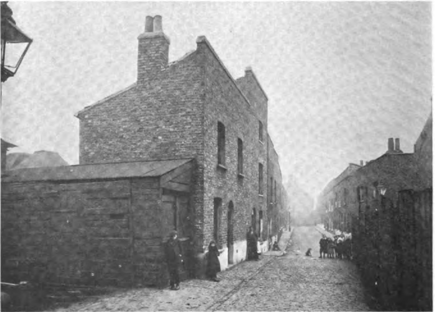
TABARD STREET AREA—VIEW, BEFORE CLEARANCE, OF FOX'S BUILDINGS
