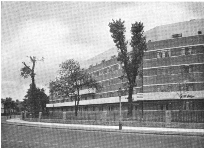
OAKLANDS ESTATE—CUBITT HOUSE
