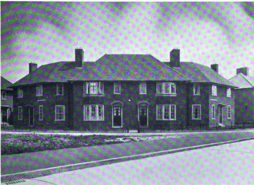
BECONTREE—JUNCTION OF LODGE AVENUE AND FITZSTEPHEN ROAD
